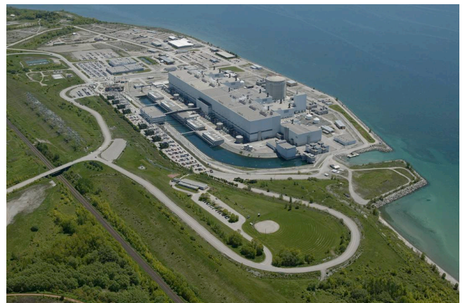
Darlington Nuclear Plant, Courtesy of Ontario Power Generation
